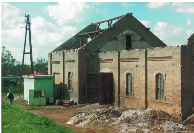
5.4: Obnova crpne stanice »Draž«, 1999. god.
